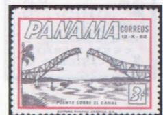
Bridge of the Americas during Construction — A140
