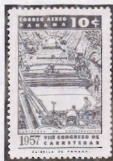
Highway Construction AP68
